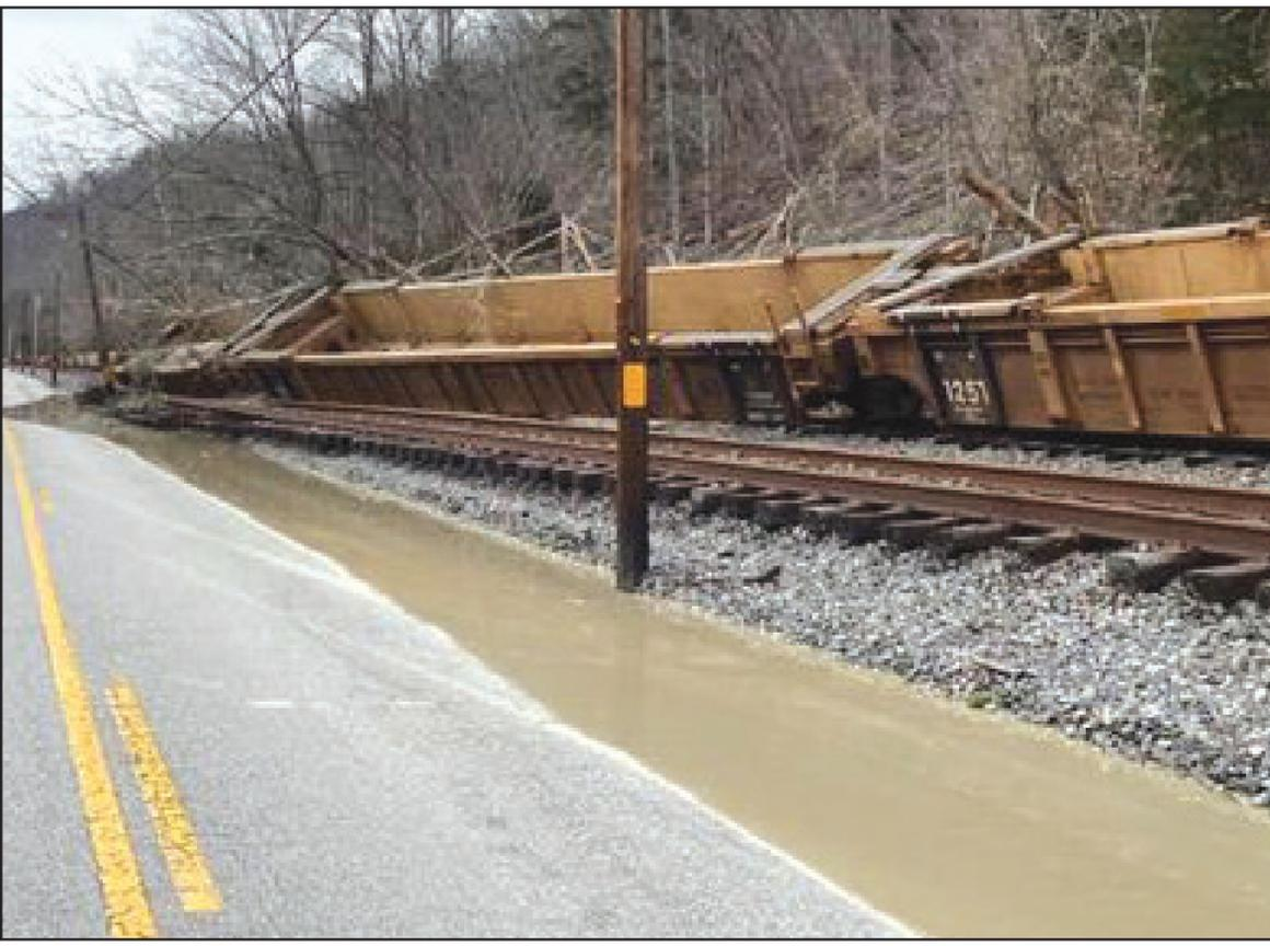
Overturned rail cars caused by a mudslide above the tracks at Millers Creek
